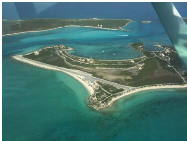
9490X on left base to an island runway
